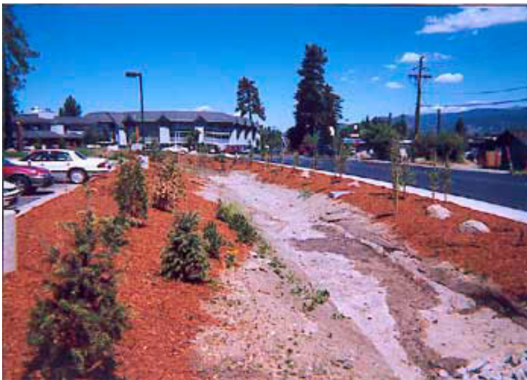
Figure 6-3: On-site Retention and Settling Basins
